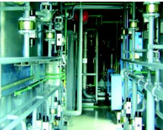
The PEM-fuel cell has taste for bio and sewage gas processed in a two-line pressure swing adsorption
