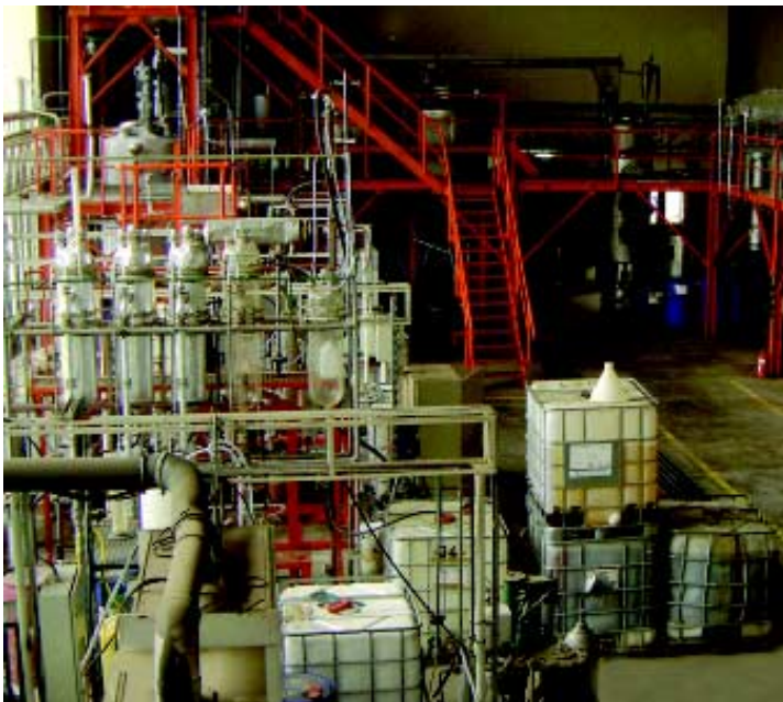
Partial view on the UDT technical shops: Pilot plants for wet oxidation of special refuse (in front) and for the extraction of natural materials (background)
